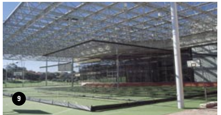
10 A15-128 Protection Nets - Fixed Net: White, 50mm square with black vinyl edging all sides. Height: as required. Cables top and bottom are fixed to the building to hold nets permanently in place.
