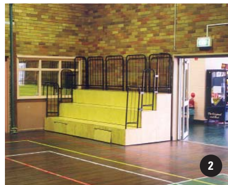
1 and 2 Continuous timber platforms with clear urethane finish
