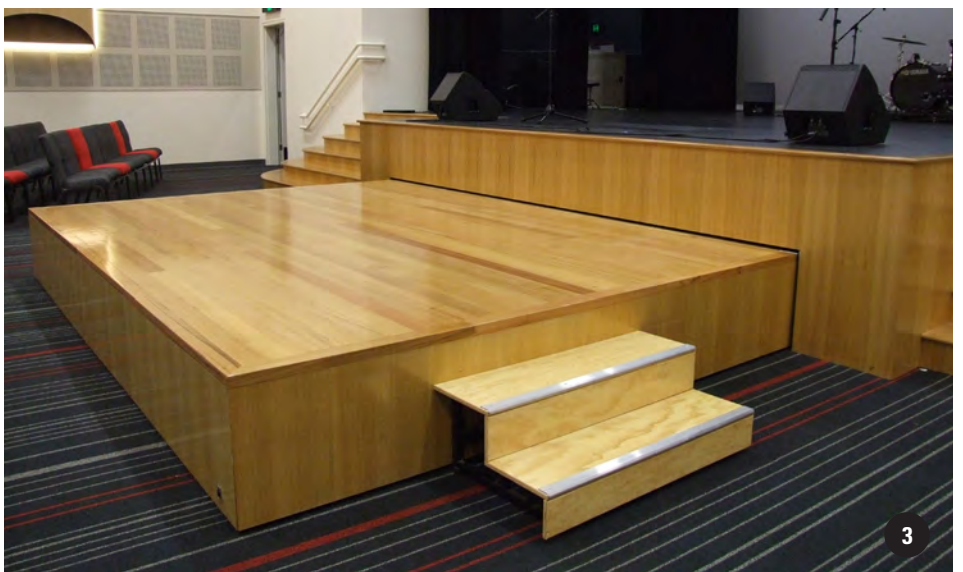
1, 2 and 3 Motorised roll out stage - stored within Height 500mm Timber finish, clear urethane
